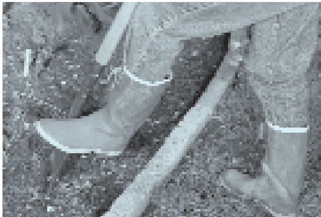
Call 811 before you dig for help in avoiding buried infrastructure.
